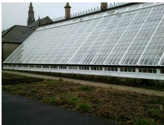
The Vinery is a lovely place. We love the cafe, and some of us have planted bulbs in the greenhouse.
